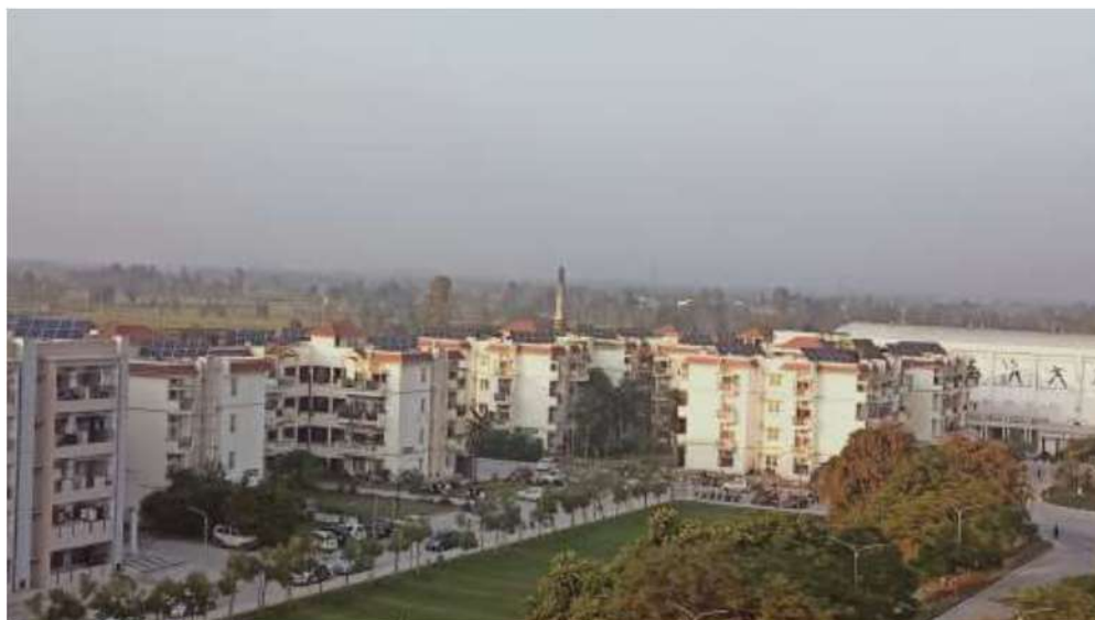
FIGURE 31: SOLAR PV PLANT
