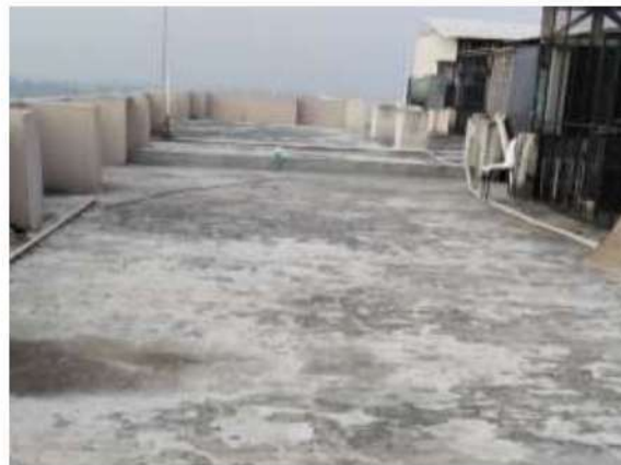
FIGURE 82: ROOF PAINTED WITH WHITE PAINT
