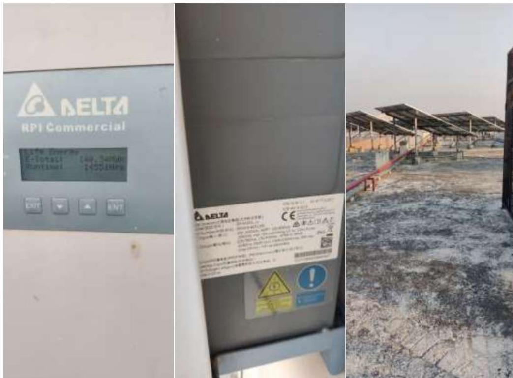
FIGURE 70: ROOFTOP SOLAR PV SYSTEM
