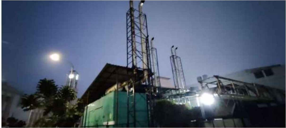
FIGURE 35: DG EXHAUST
