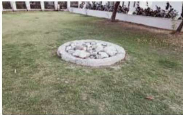
FIGURE 18: RAIN WATER HARVESTING PIT
