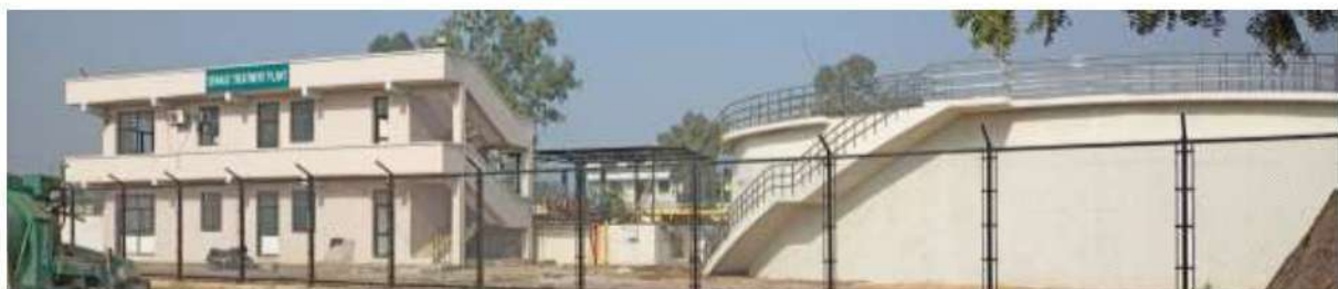
FIGURE 19: SEWAGE TREATMENT PLANT
