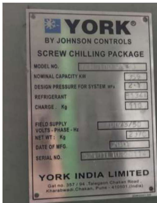
FIGURE 43: CHILLER R-134A REFRIGERANT
