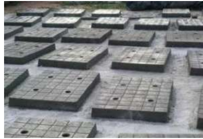
Figure-2:- Solid precast slab
